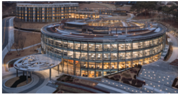
Solar panels installed in the LifePark Training Center
